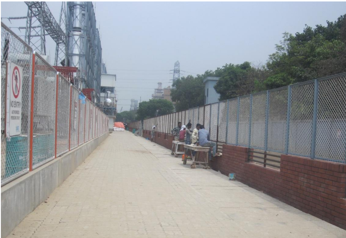
Figure 6-1: Paved View of the Plant Premises
