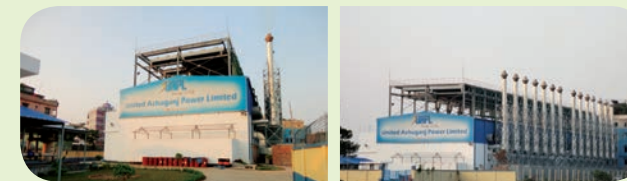
United Ashuganj Power Limited
